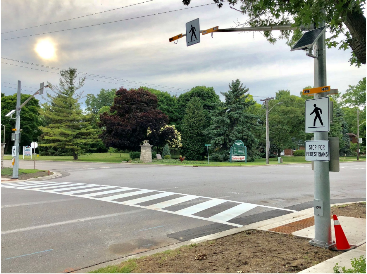
Photo: Pedestrian crossover at Canatara Park.
