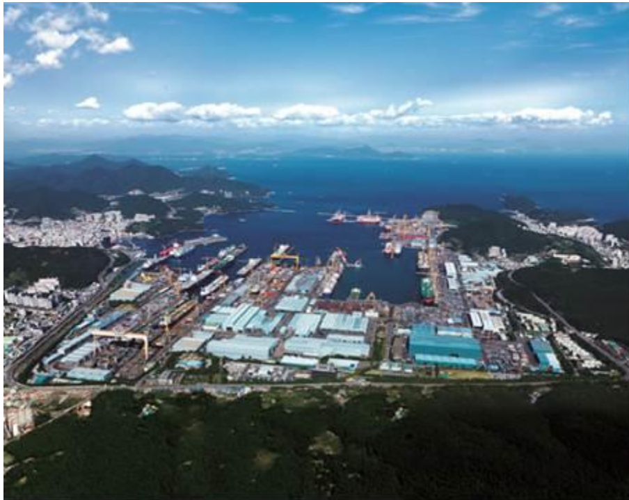
Figure 5-10: Daewoo Fabrication Yard, Korea
