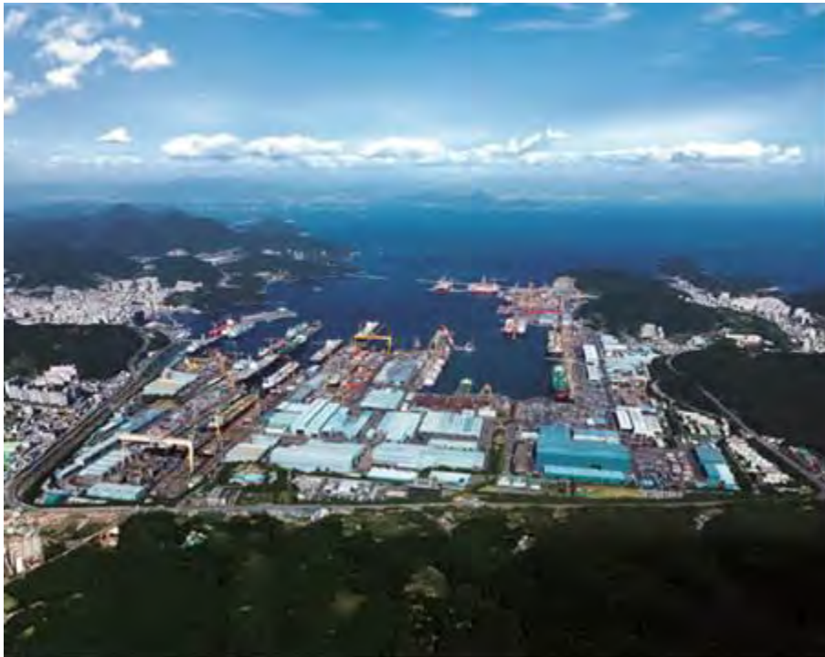
Figure 5-10: Daewoo Fabrication Yard, Korea
