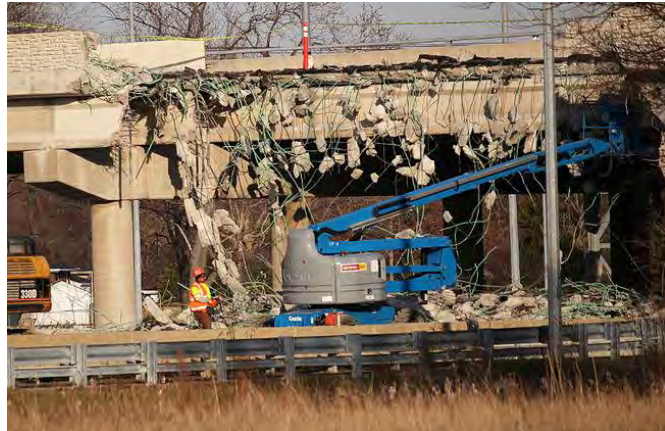
Figure 2-1: Repairs to Hwy 402 Bridge from Oversize Vehicle
