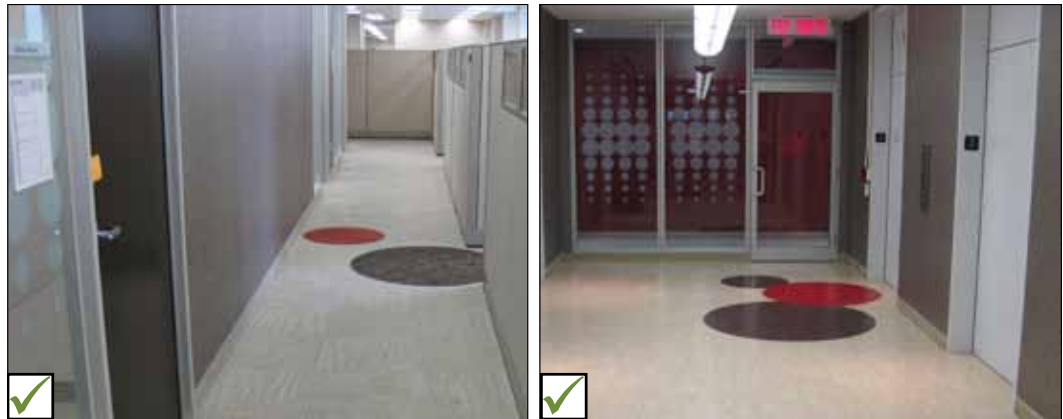
Example of floor surface and elevator door finishes that minimize glare.
