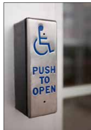
Example of rectangular shaped power door operator control to be used for retrofit situations only.
