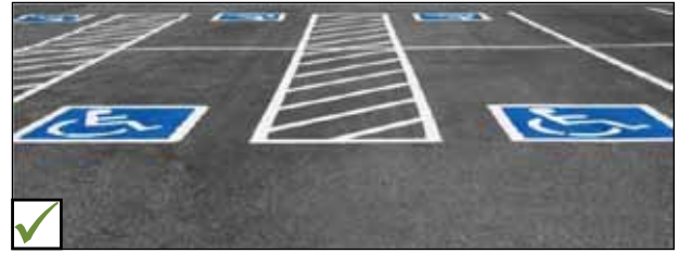
Accessible parking spaces with shared access aisle. Source: Taken from "Illustrated Technical Guide to the Accessibility Standard for the Design of Public Spaces" by GAATES, 2014, p. 123.
