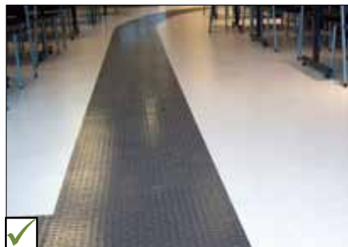
Example of tactile floor surface to guide users with vision loss (Best Practice).
