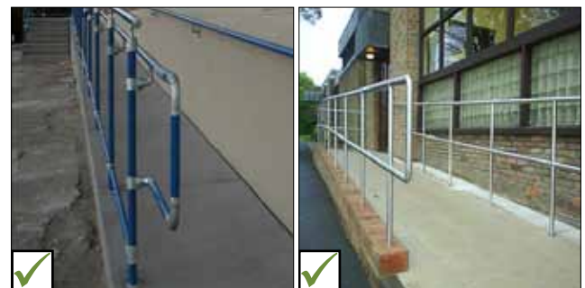
Figure 7b: Handrail Returns to Wall
