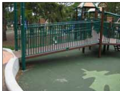
Ramp connected to elevated play components.
