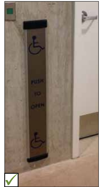
Example of large vertical extended power door operator control.
